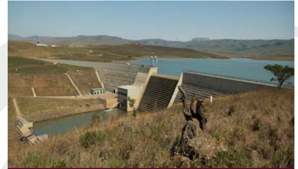
Ingula Pump Storage
